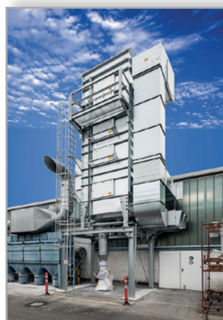
Schuko filter system especially for carbon dust extraction; Photographer: Rainer Bez
